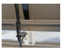
• **Repair, Safety Issue:** The overhead garage door is damaged and needs repair. The garage door opener did <u>not</u> automatically reverse under resistance to closing. *There is a serious risk of injury, particularly to children, under this condition.* This should be dealt with immediately. The opener may need replacement.
