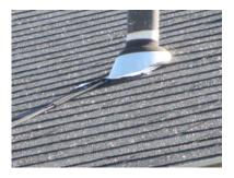
• **Monitor:** The skylight flashing should be carefully monitored. Skylight flashings are extremely vulnerable to leakage, and all skylights will leak in time. Generally, those with the highest sides are the easiest to install in a weathertight fashion.
